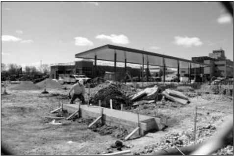
The Sheetz gas station on Navarre near St. Charles is shown under construction.
