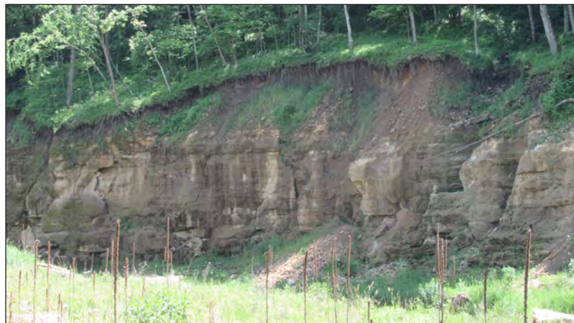
Sandstone cliffs remain where a Coon Creek Watershed flood control dam failed during August 2018's catastrophic flooding. Following the flood, the Natural Resources Conservation Service issued an unprecedented, formal recommendation to decommission all 14 of the watershed's aging flood control dams. Photo by Rebecca Lave.
