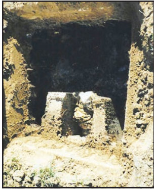
Deteriorating Concrete Inlet Baffle
