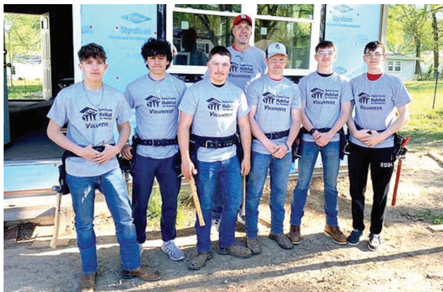
Pictured are morning DCTC Construction students who helped with the building. CONTRIBUTED PHOTOS
