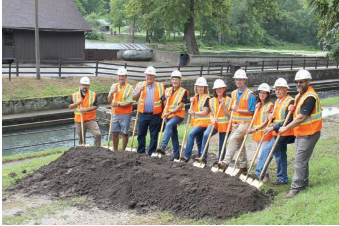
Groundbreaking begins the construction phase of the renovation project at MDC's Bennett Spring Hatchery. Fishing will continue with minimal disruption at Bennett Spring State Park throughout construction. REFLEX PHOTOS BY JOY BEAMER
