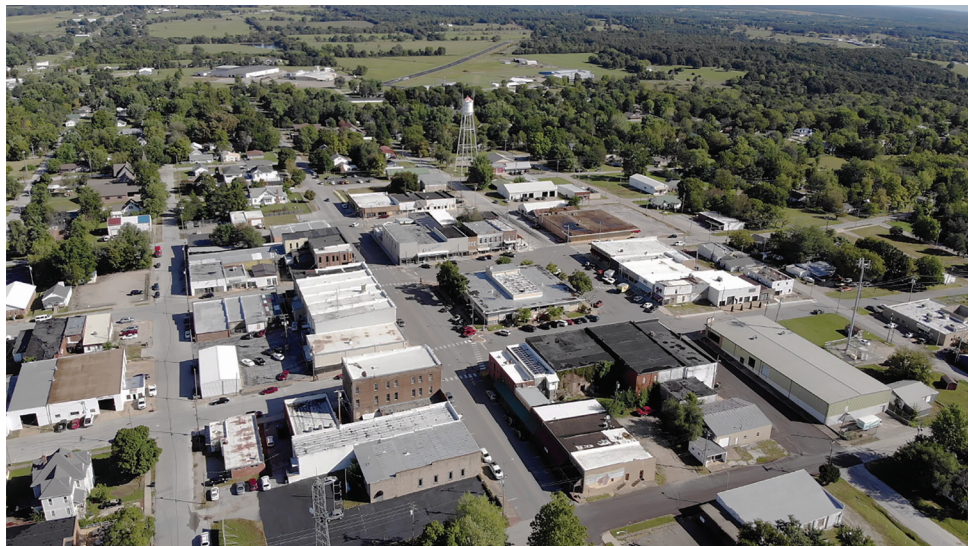
This aerial view of Buffalo was taken before the replacement of the old water tower with the new one. CONTRIBUTED PHOTO
