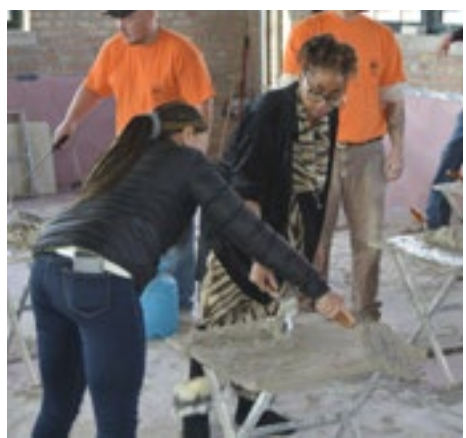
Students check out rebar work at the Iron Workers Local 395 display (top). Students learn about mortar and bricklaying with members of Bricklayers and Allied Craftworkers Indiana/Kentucky Local 4 (bottom).
